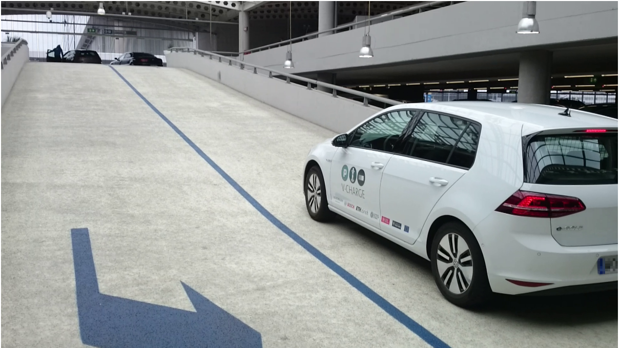
Figure 25: Ramp at the Schiphol Excellence Parking garage in Amsterdam, connecting levels 2 and 3.
